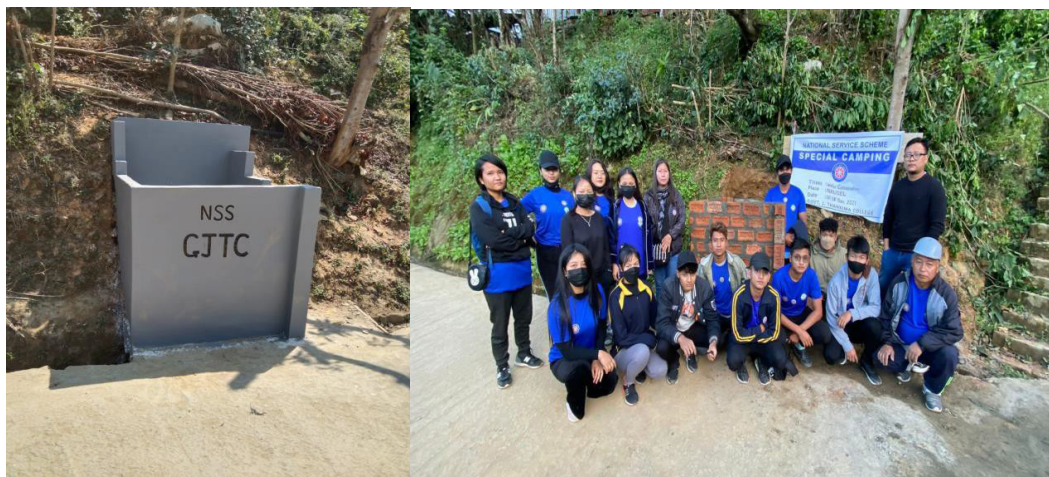
Pic 5 : Construction of Public Urinal, special camp at Nausel
