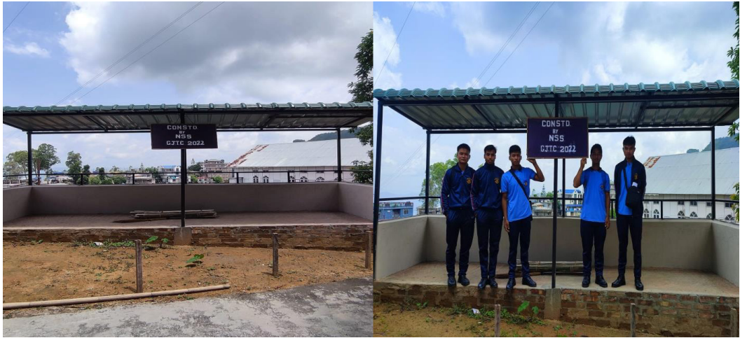
Pic 6 : Construction of Rest Shed, special camp at Central Campus Bawngkawn
